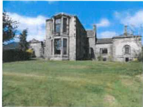
South elevation of Urquhart Farmhouse
